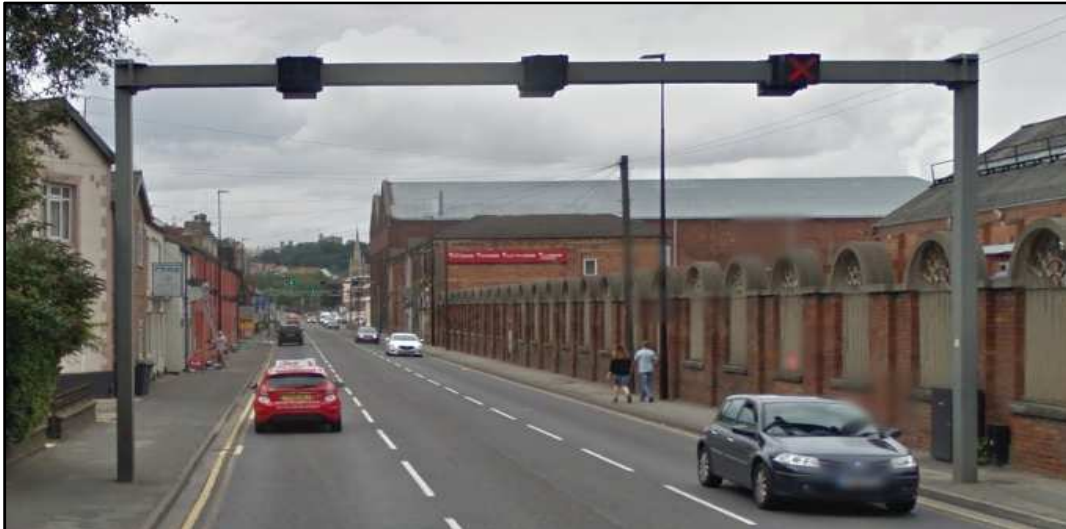
Figure 2: Northbound view of A15 Canwick Road
