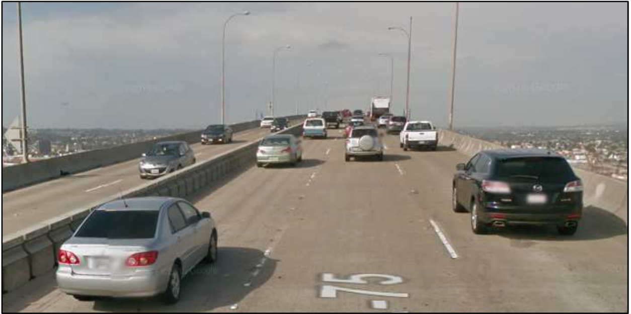
Figure 5: Northbound view of CA-75 on the Coronado Bridge
